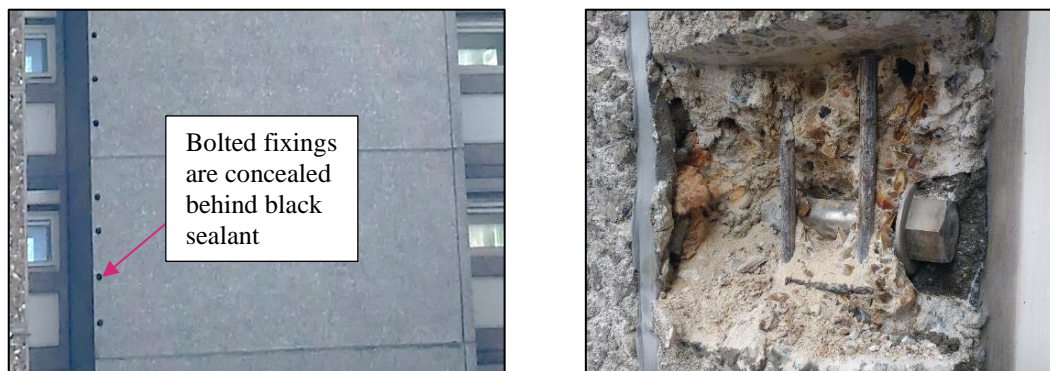
Figure 10 Fixings bolts are concealed behind black sealant (LHS). Fixing bolt exposed by breaking away surrounding concrete (RHS)
